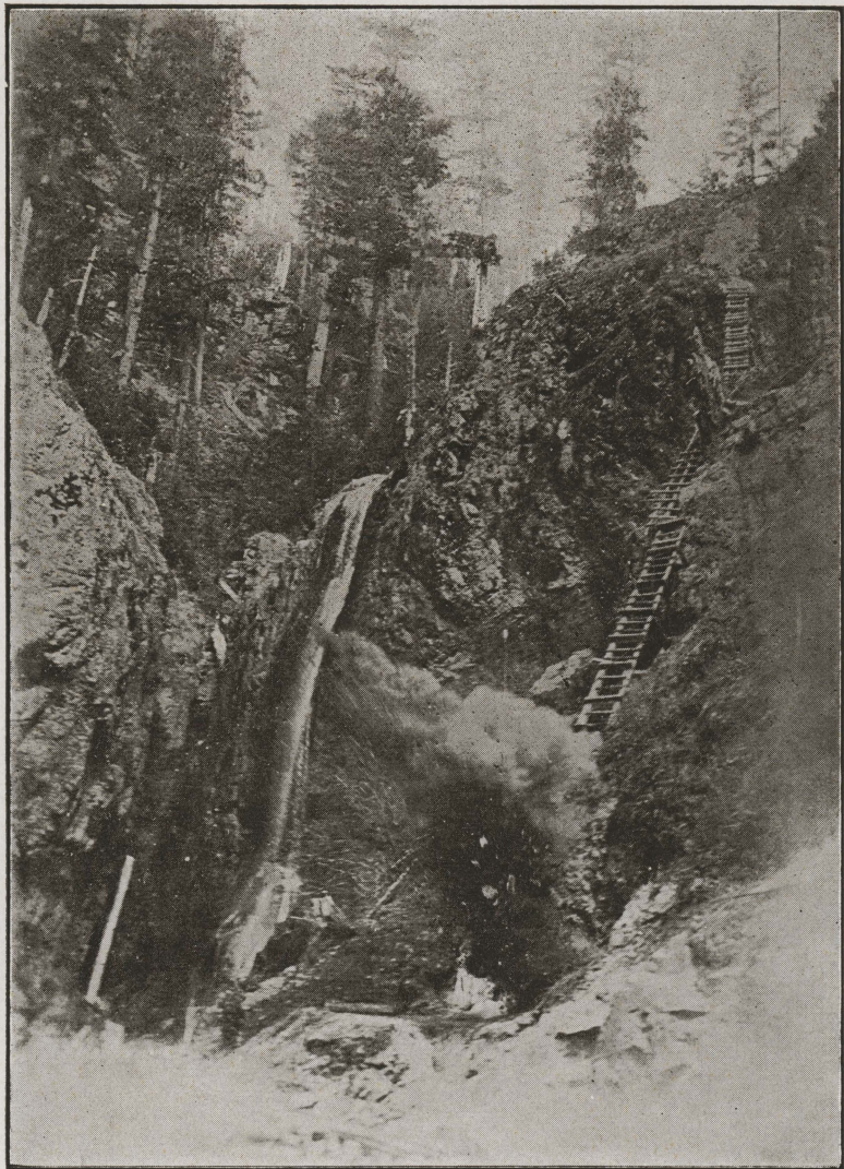
Silver King Falls, location of power site, giving ample power for all purposes. Blasting location for plant.
