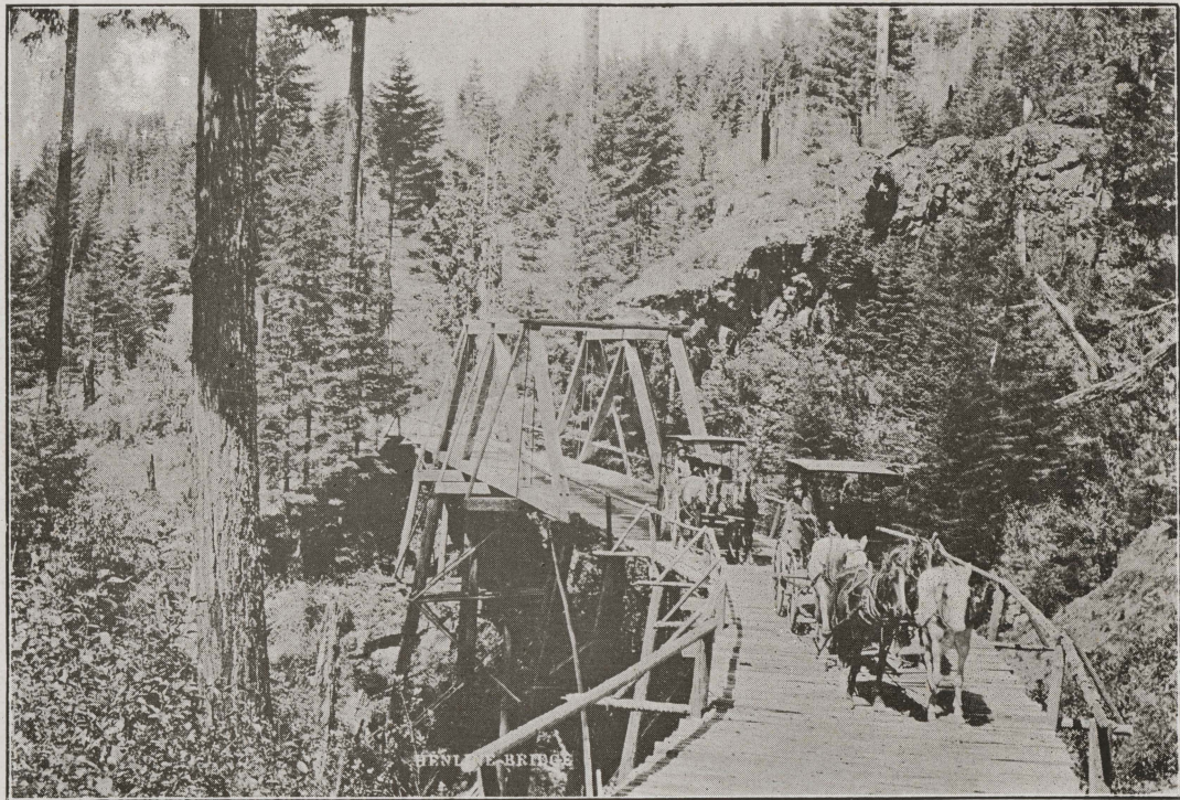
Bridge crossing Henline Creek, approaching Silver King Mine, showing good transportation.
