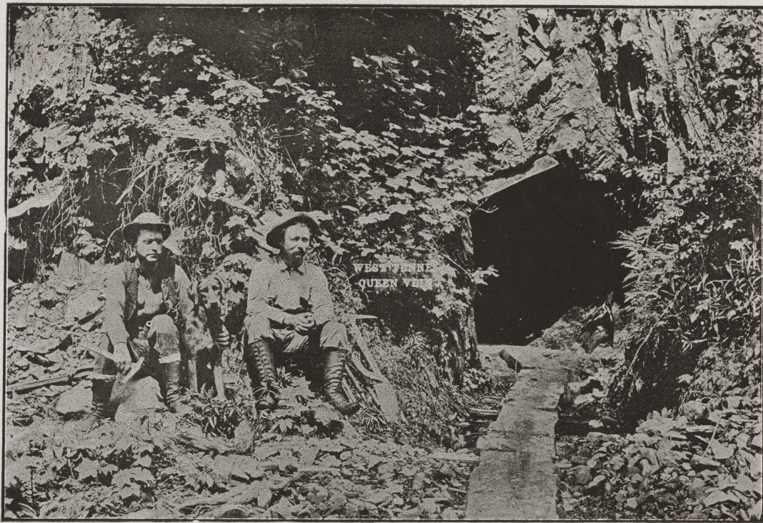
West Prospect Tunnel on Queen Vein. The face of this tunnel is 300 feet from face of East Tunnel, all showing ore-bearing formation.
