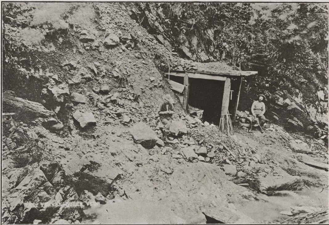
East Prospect Tunnel on Queen Vein, showing ore formation, width from hanging wall to foot wall about 130 feet.
