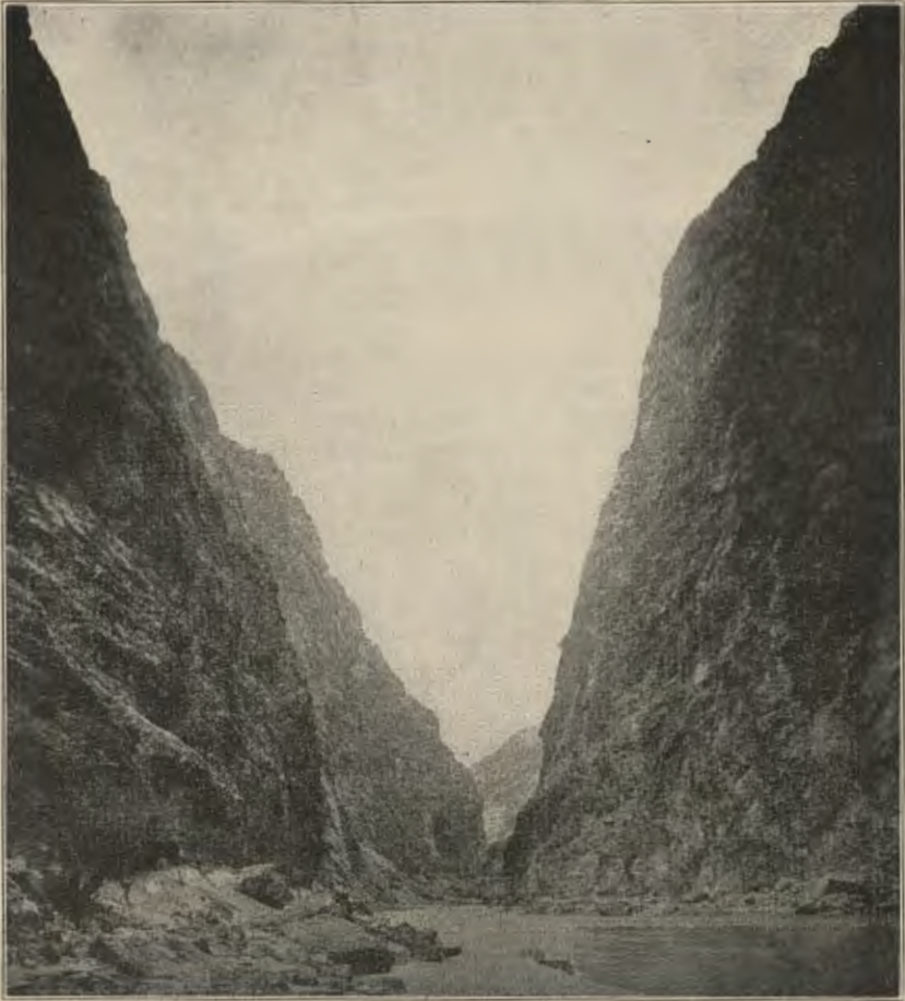
BOULDER DAM SITE
