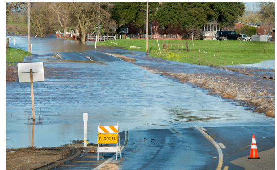
Flooding near Elk Grove, Calif. during record rain year 2017
