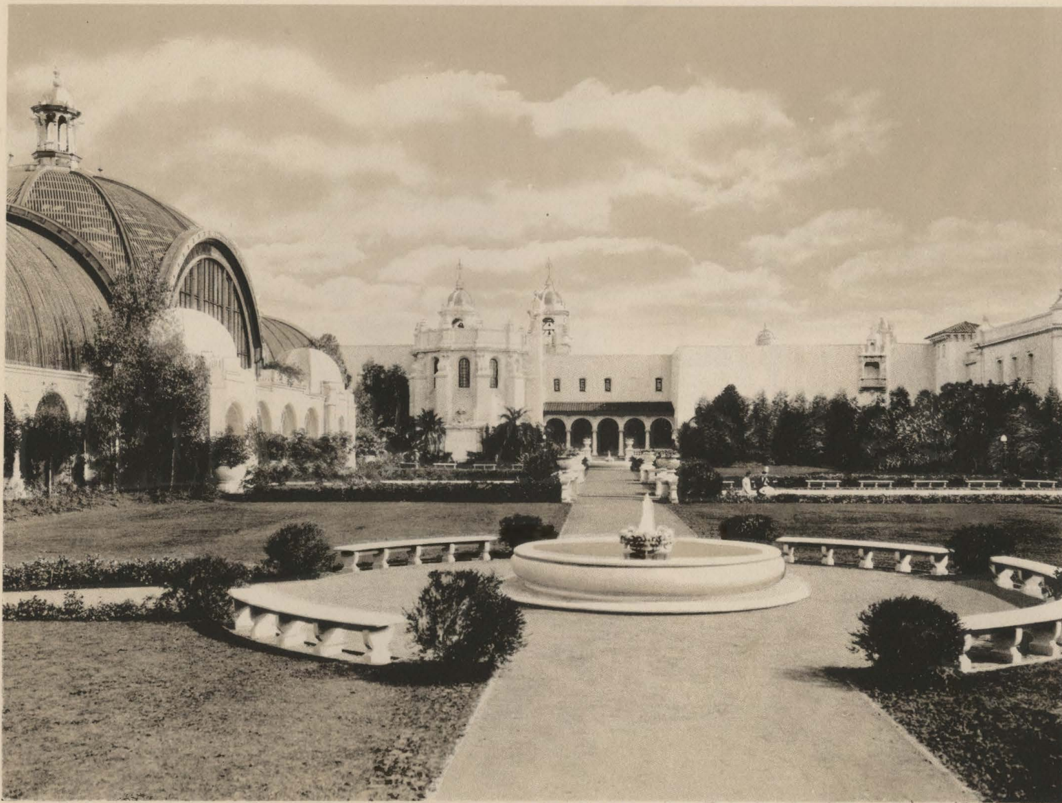
The Botanical Gardens showing Botanical Building on the left and Varied Industries Building in the Center, Panama-California Exposition.
