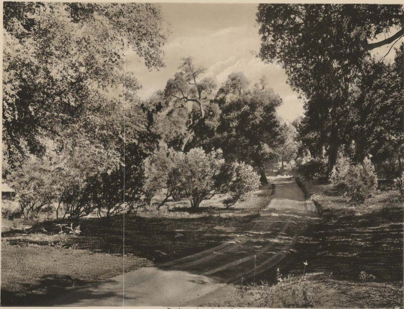
Roadway through the Oaks.
