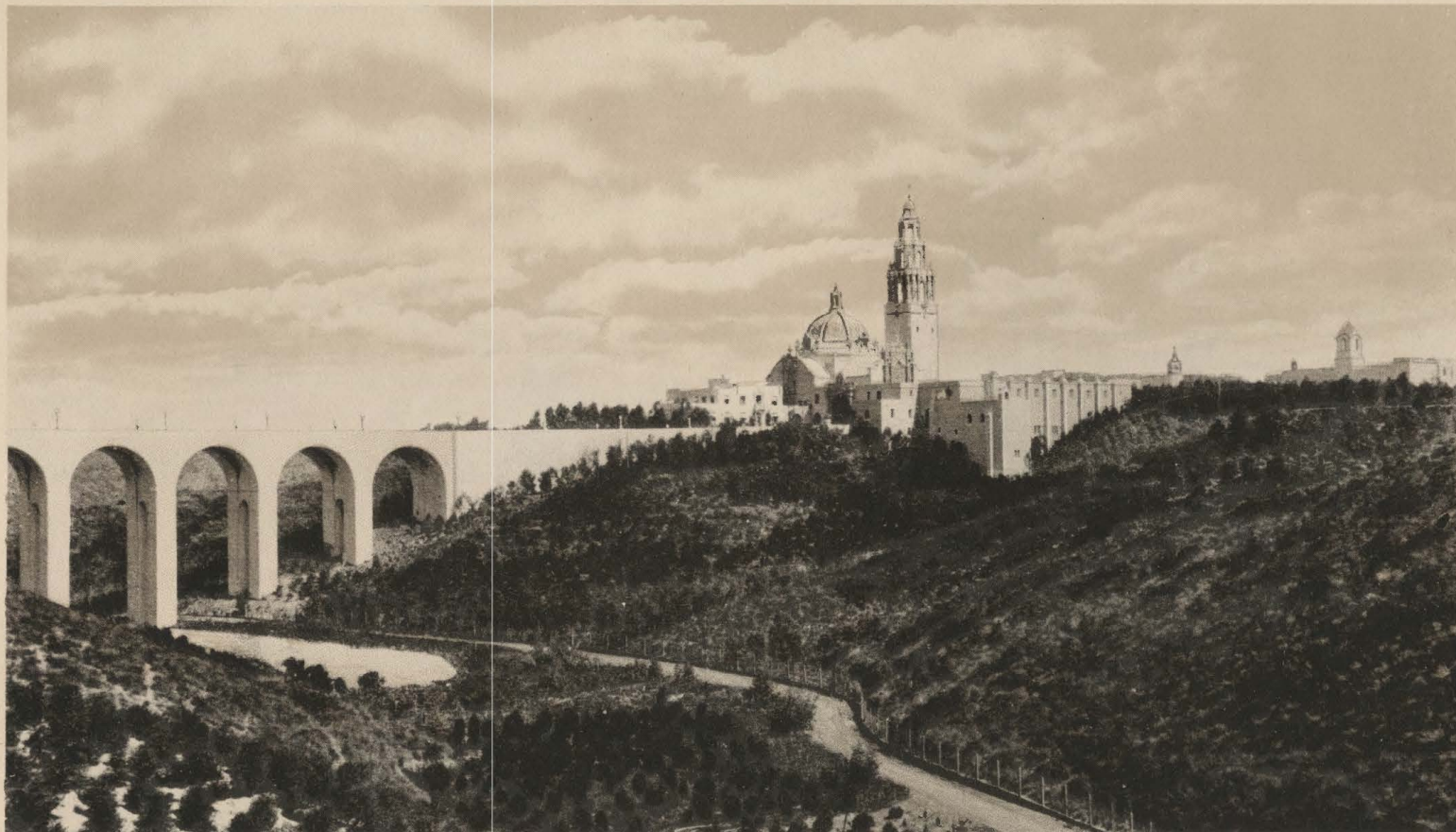
Puente Cabrillo across Canyon, West approach to the Panama-California Exposition, San Diego, Cal., Jan. 1st-Dec. 31st, 1915.
