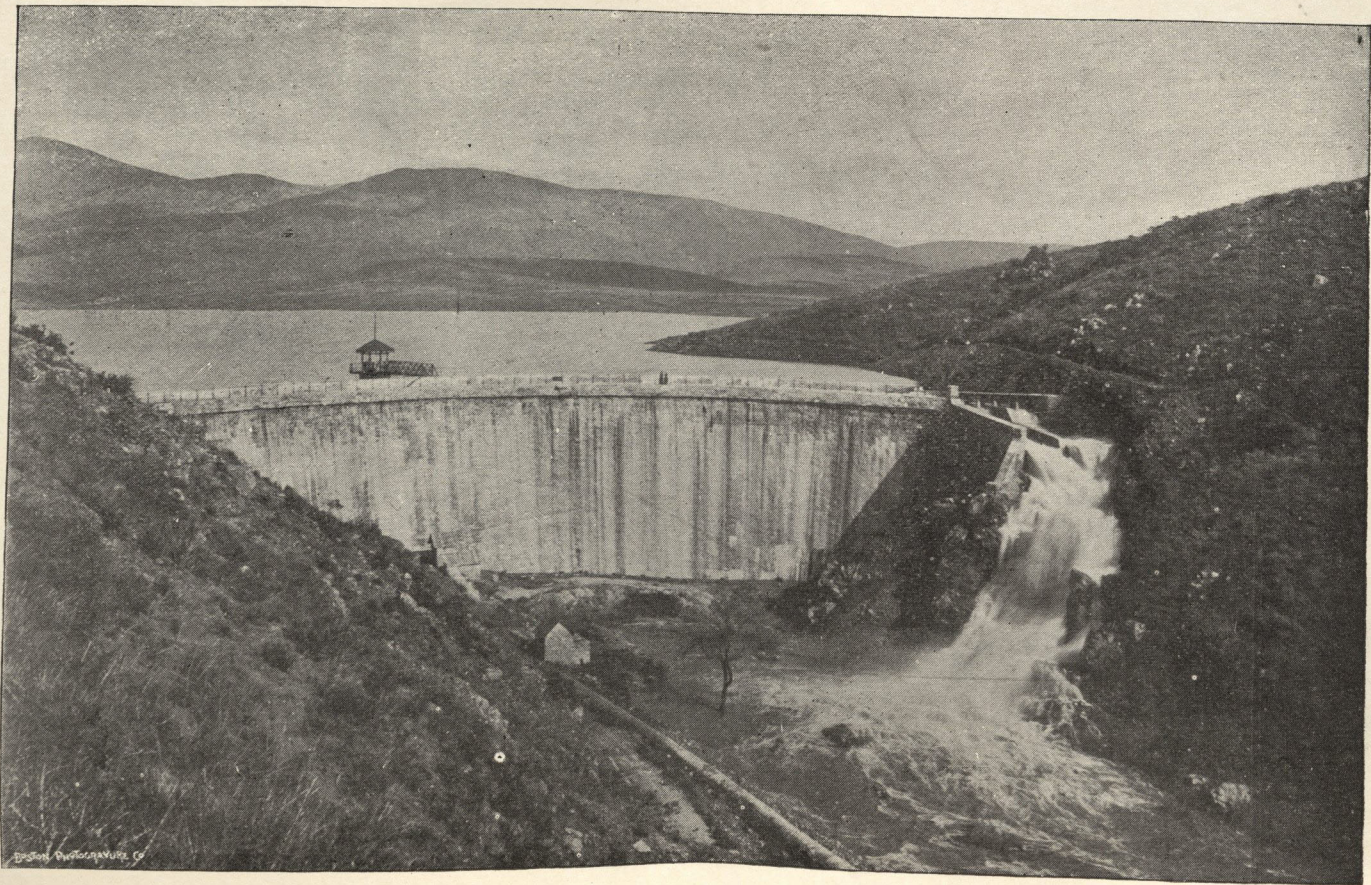
THE SWEETWATER DAM, BUILT AND OWNED BY THE SAN DIEGO LAND AND TOWN CO.
