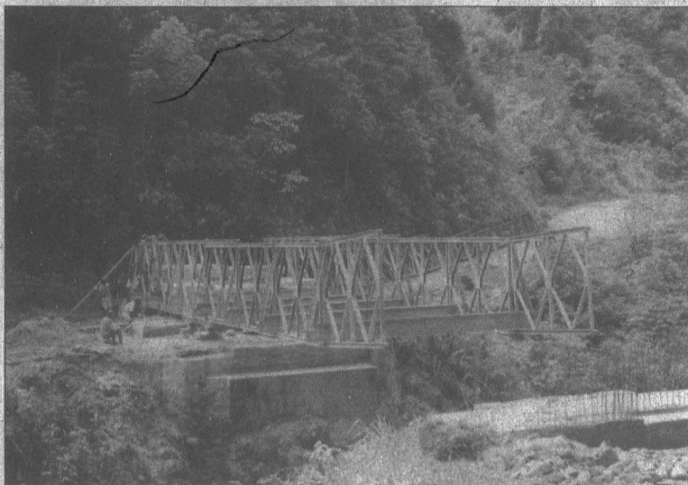
Construction of the Kapau bridge under the Yumi Yet Bridge program.
