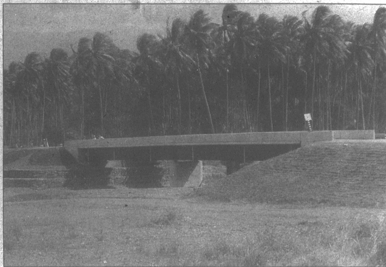
Bijita bridge located on the Highlands highway.
