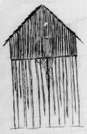
House seen at WOIBI 26/4/57. First of type struck. Roof of sago thatch. Dimensions; from ground to floor 12 feet; from floor to ridge 8 feet. 12 feet wide and 20 long. Timber used throughout no larger than mans arm. Interior lined with bark. Exterior walled in split billets of timber. Woven wicker basket hanging underneath contains clay. Used as fireplace.
