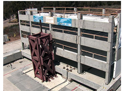
Precast concrete building
