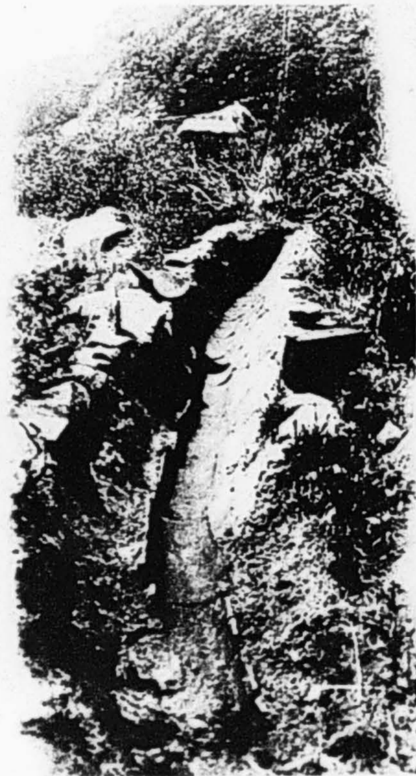
Section of the Old Mission conduit uncovered near Mission Gorge gaging station. Practically intact after 125 years. Also, a view of the right wall of a broken section, showing mortar plaster.
