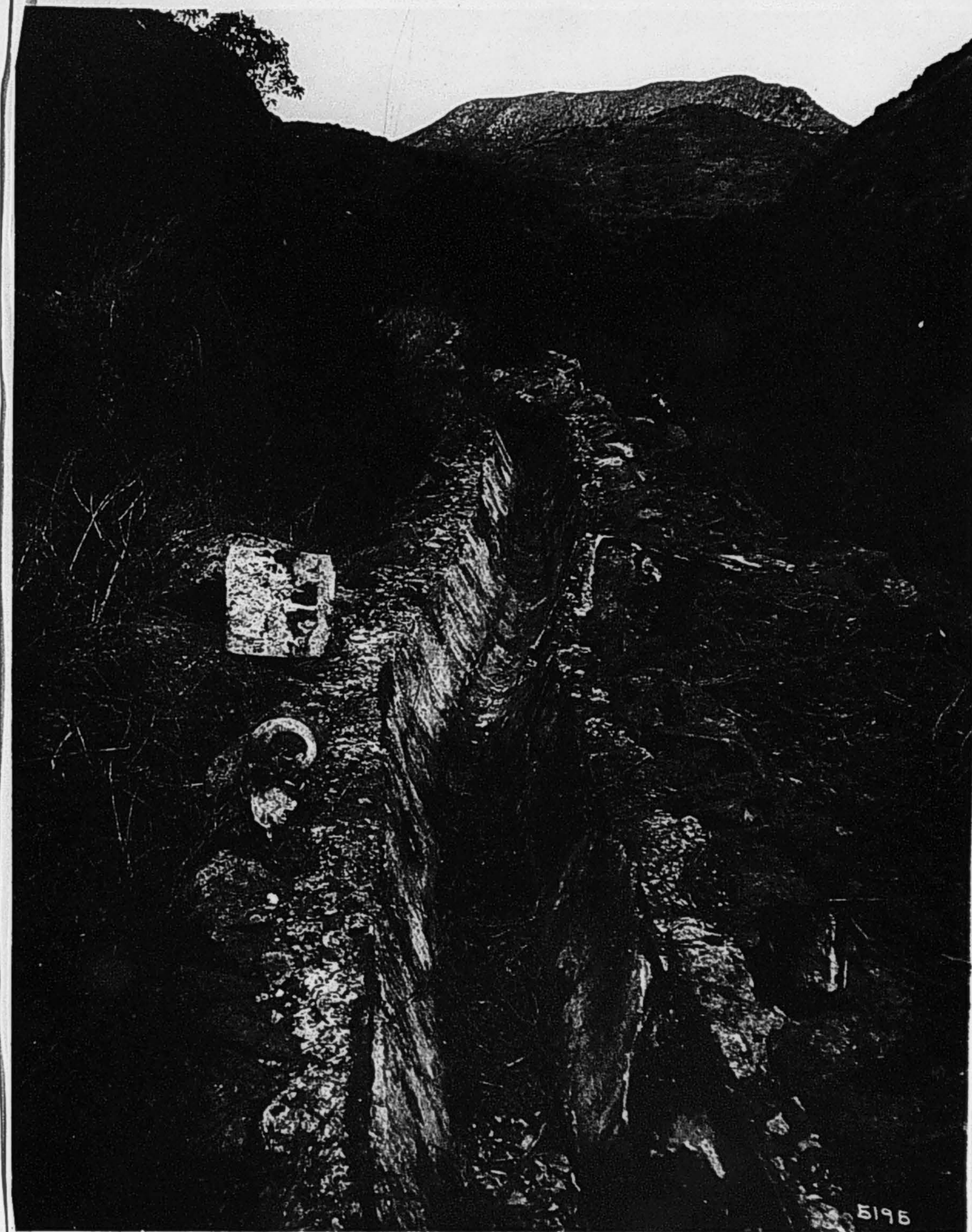
Section of Old Mission conduit practically intact, showing tile sides and bottom.
