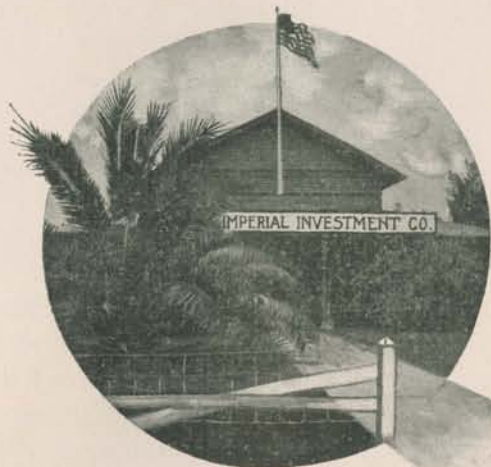
OFFICE OF IMPERIAL INVESTMENT CO., BRAWLEY, CAL.
