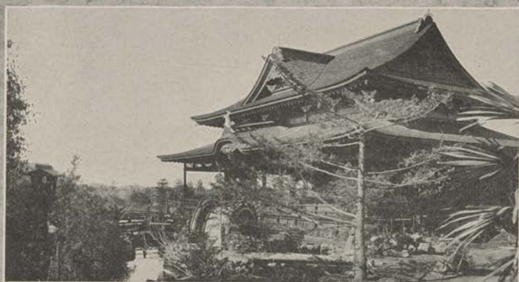
ACROSS THE LAWN BY THE MODEL CALIFORNIA BUNGALOW BUILDING OF INTERNATIONAL HARVESTER CO. OF AMERICA IN THE JAPANESE GARDENS—JAPAN AND FORMOSA BUILDING
