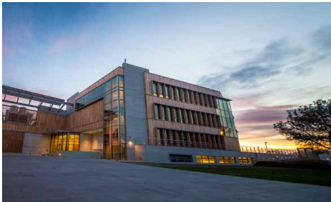
Craig Venter Institute research facility on the UC San Diego campus was designed to exceed requirements for LEED Platinum certification and to be carbon neutral.
