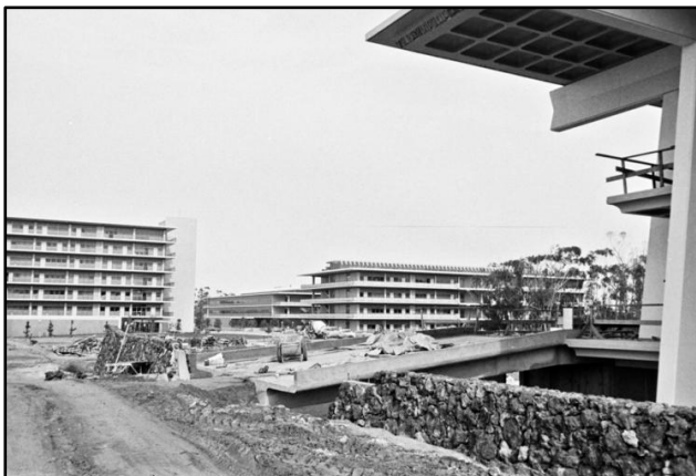
First College under construction - 1964-65
