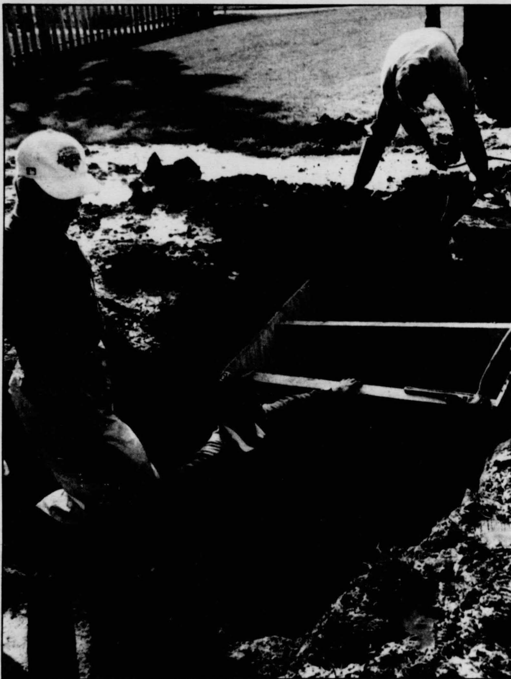
Construction workers search for a break in the water main outside Beagle Hall Wednesday. Revelle dorms were without cold water for much of the day.
