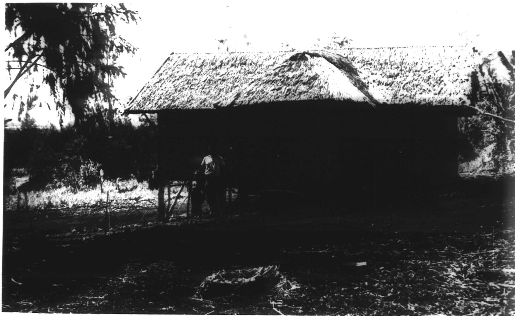
Plate 9. A house of 'modern' style, designed by the owner, and built of traditional housing materials - woven cane grass walls and thatched roof of Imperata .
