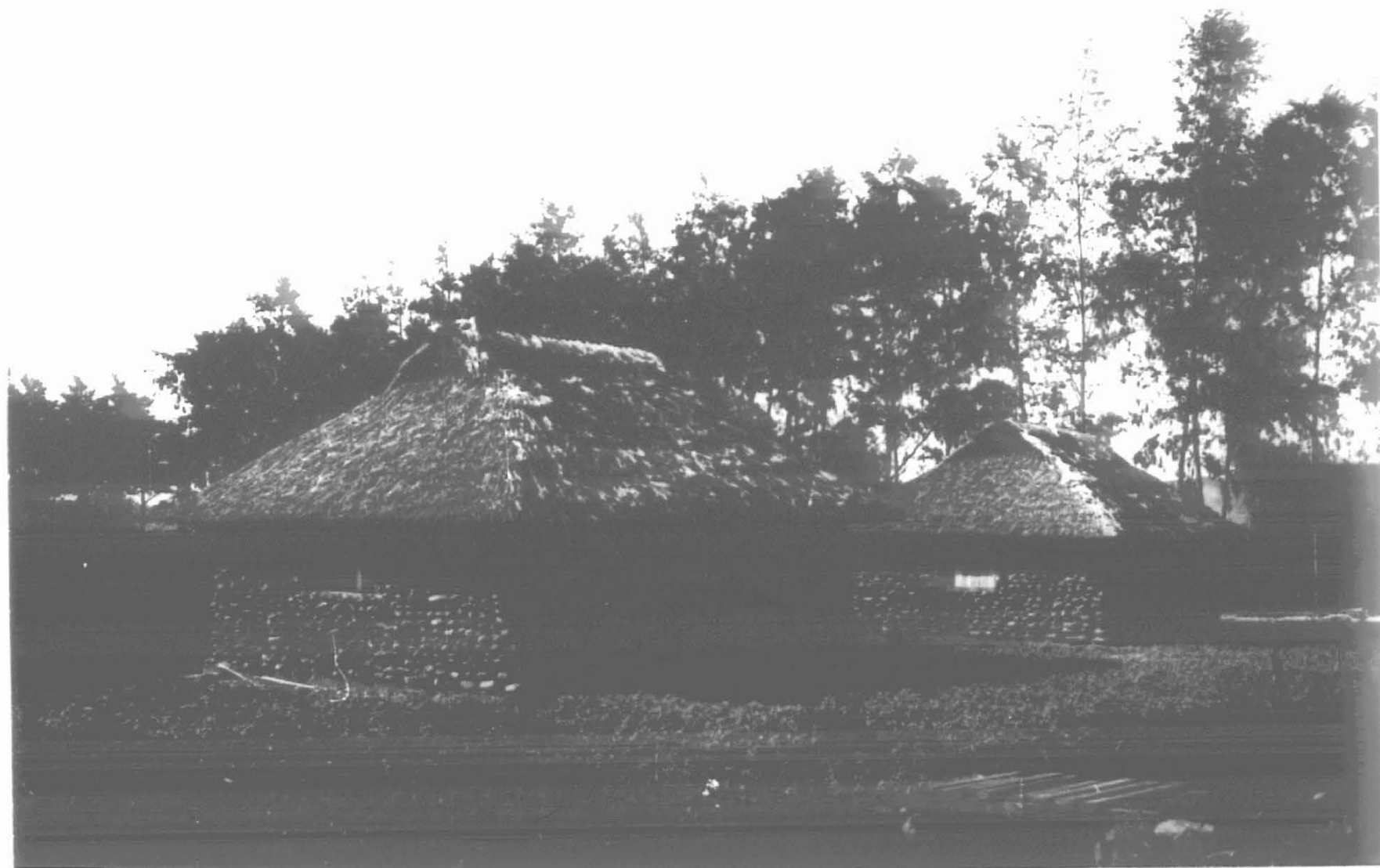
Plate 64. Houses for plantation labourers, constructed of stones from river beds. Housing of this standard is rare on plantations, although inexpensive to construct.
