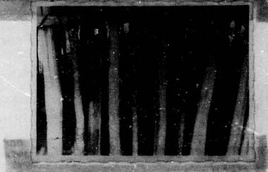
Looking through the walls of a partially constructed house. Note the slightly raised floor and provision for fire place.
