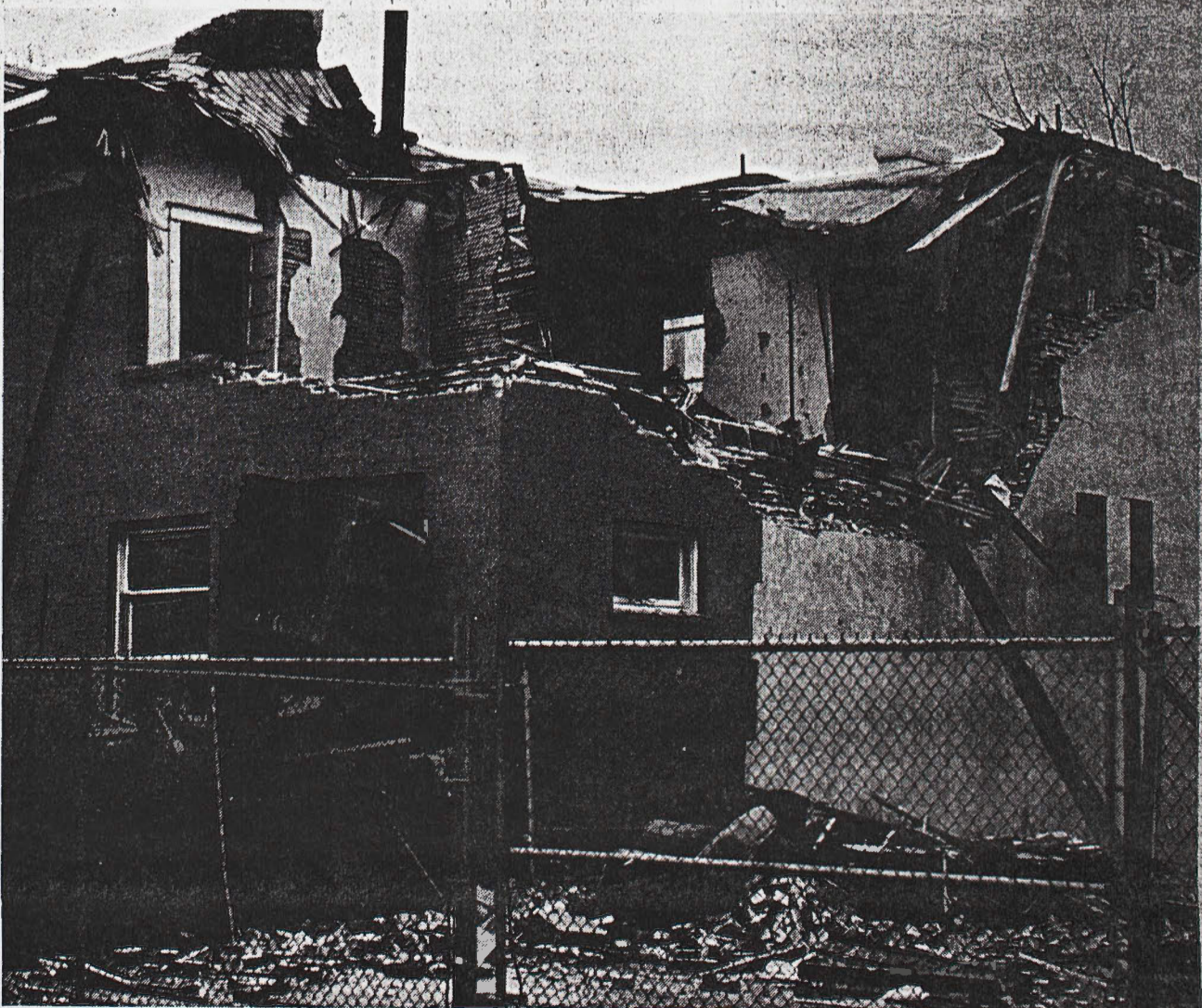
There was an explosion at dormitory of Escuela Tlatelolco during March 17, 1973, police attack. Cops said dynamite stored in building caused blast but then demolished remains of the building a day later, destroying all the evidence.
