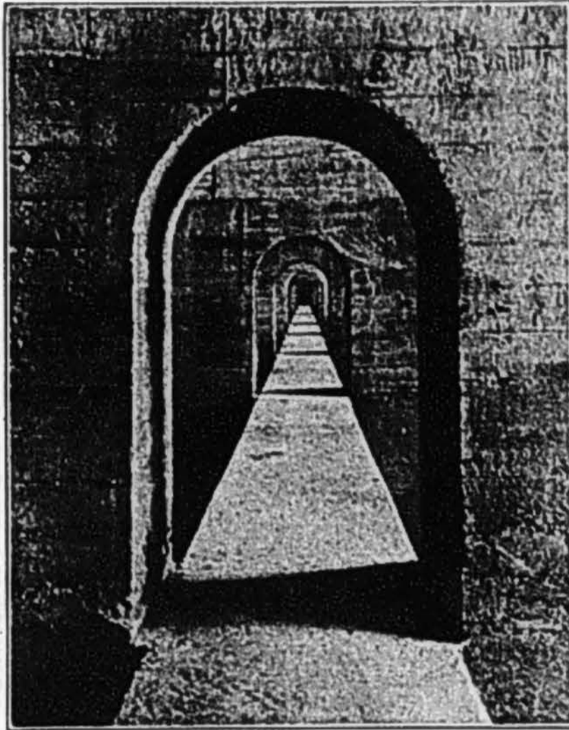
CONCRETE WALK IN DAM
