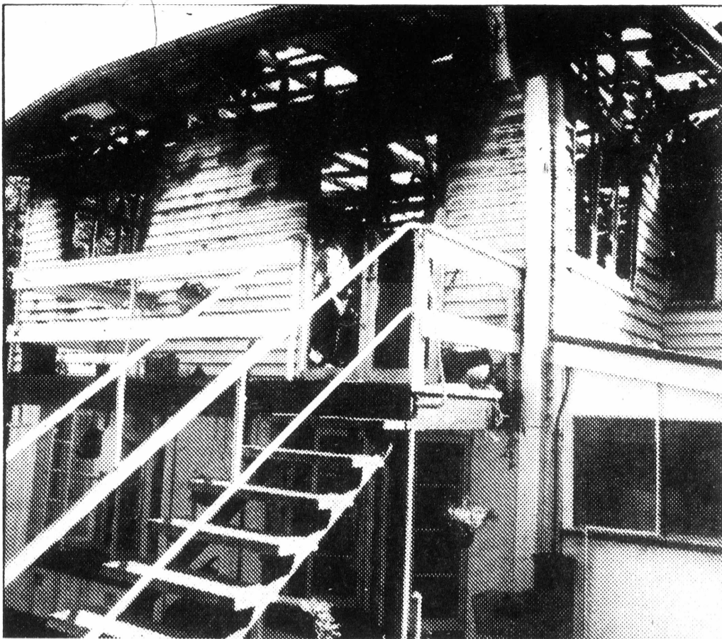
• Hostel bilong ol olpela paitman bilong woa long Toowong, Australia em paia i bin kukim long Sarere 27 Julai, 1991. Nogat wanpela man i indai o bagarap. Tasol ol i lusim olgeta samting bilong ol. Ripot i tok masin bilong hotim ges i mas kamapim dispela paia.
