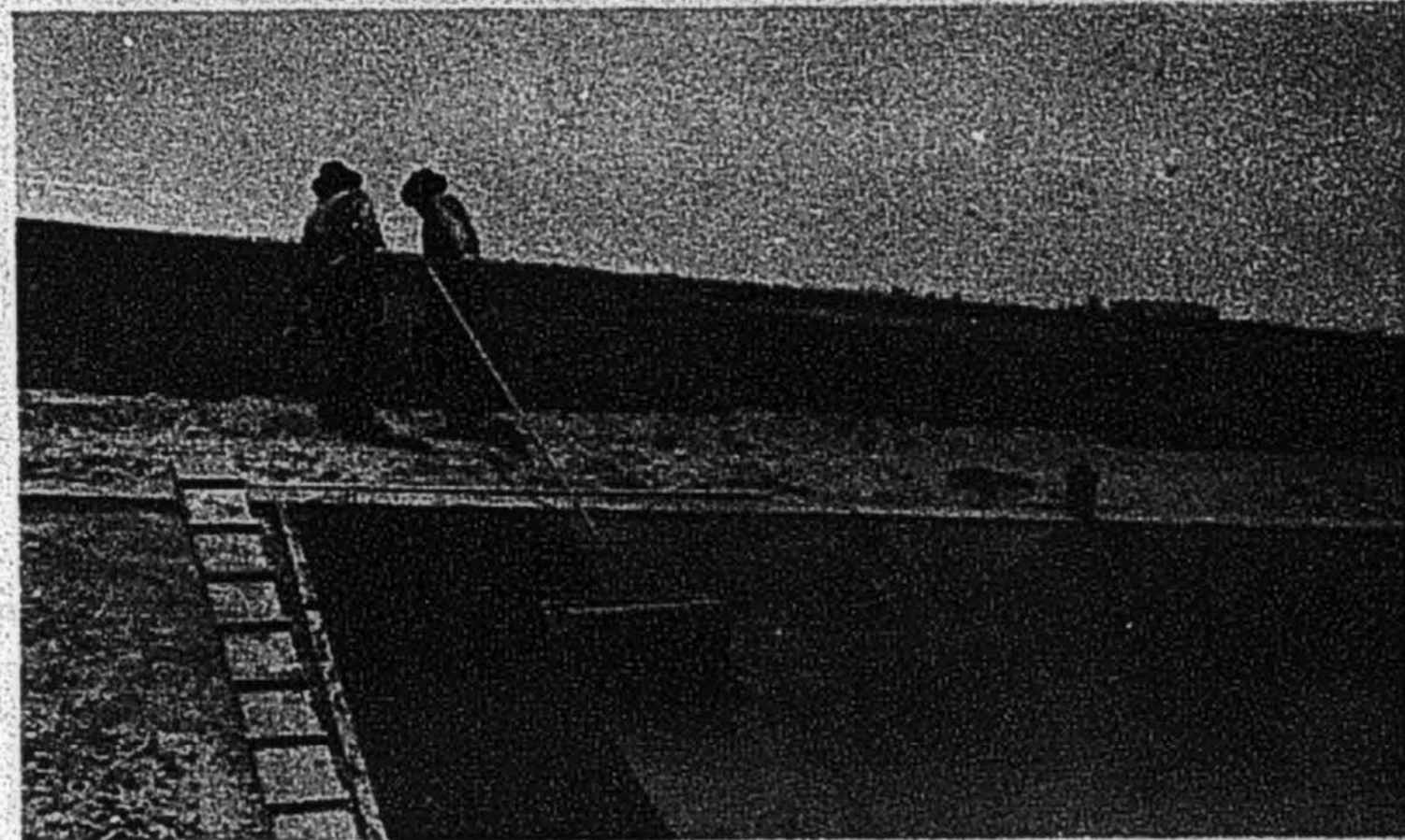
The mixture was rich enough in asphalt to seal up thoroughly under the compression afforded by a light hand-roller
