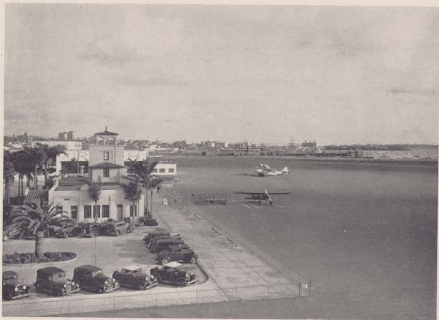
Administration Building at Lindbergh Field. The municipal piers and waterfront area of San Diego may be seen in the background.
