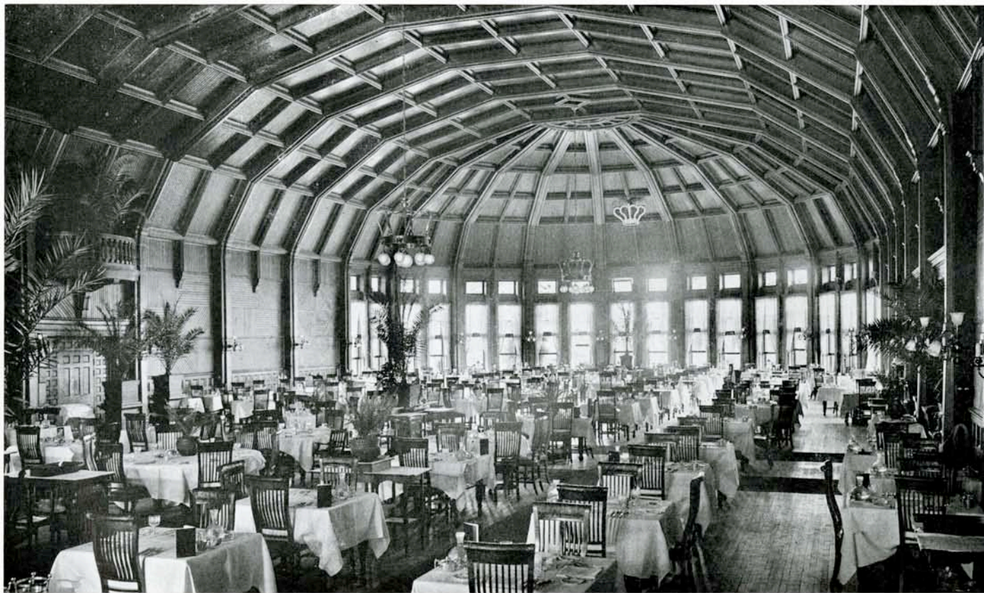
SOUTH END OF DINING-ROOM
