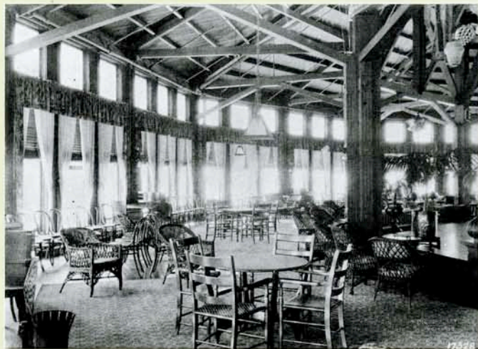
SUN PARLOR ALMOST SURROUNDS LARGE BALLROOM
