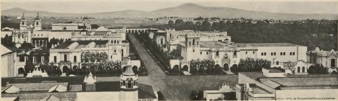
LOOKING DOWN THE PRADO FROM THE CALIFORNIA TOWER
