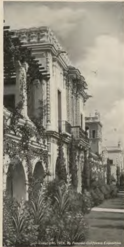
WEST FACADE, HOME ECONOMY BUILDING
