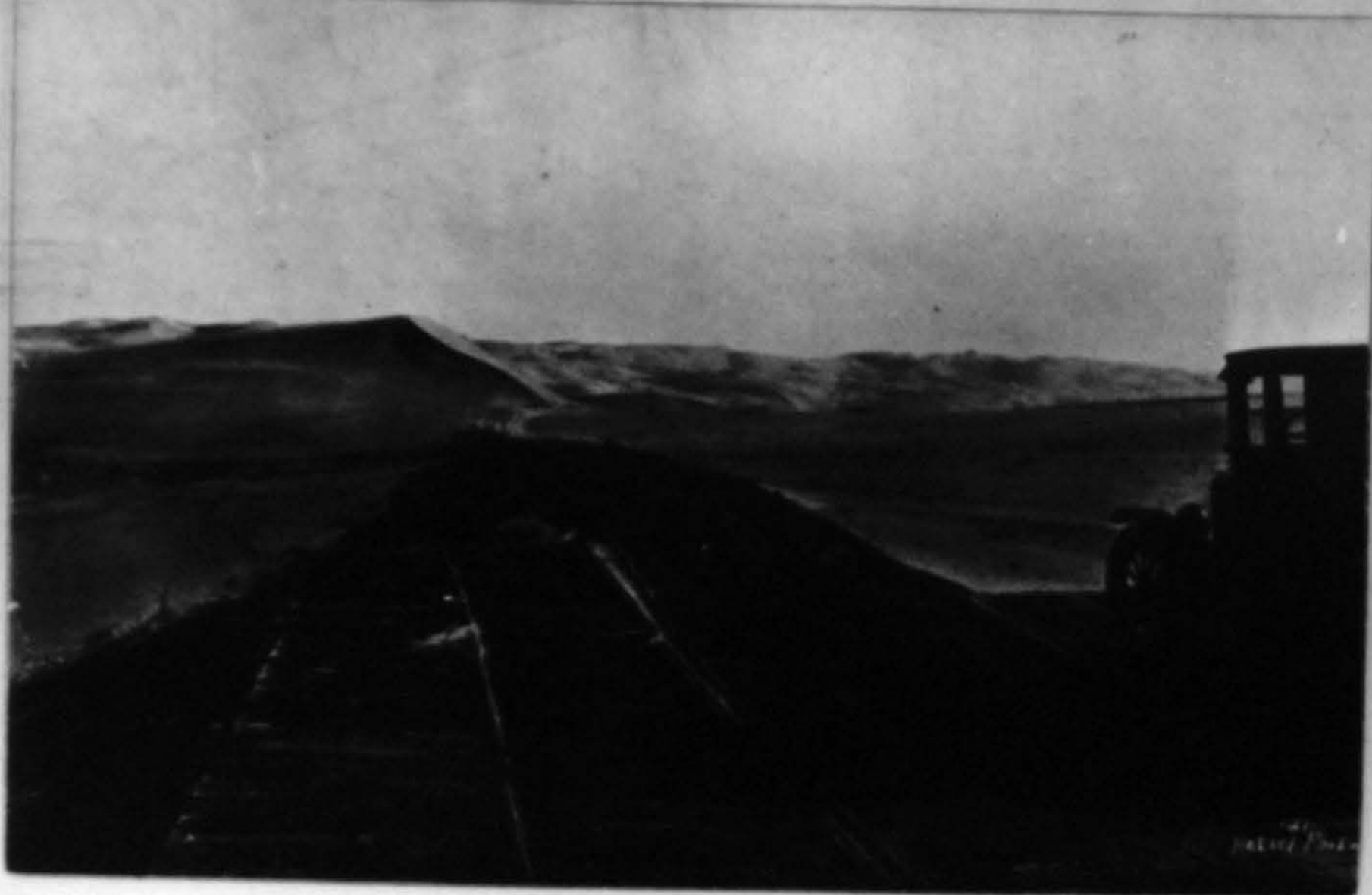
Sand Hills, Imperial County.—A turn-out on the old plank road. The rapid deterioration of this road and the hazard to traffic because of its narrowness, were the reasons for its replacement by a permanent asphaltic concrete pavement.
