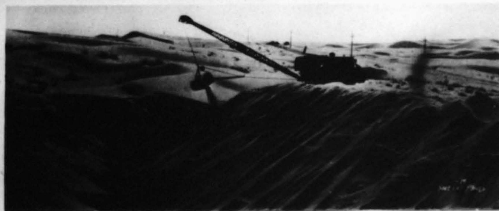
Sand Hills, Imperial County, California.—Drag-line scraper at work constructing fill for new asphaltic concrete pavement across the Sand Hills.
