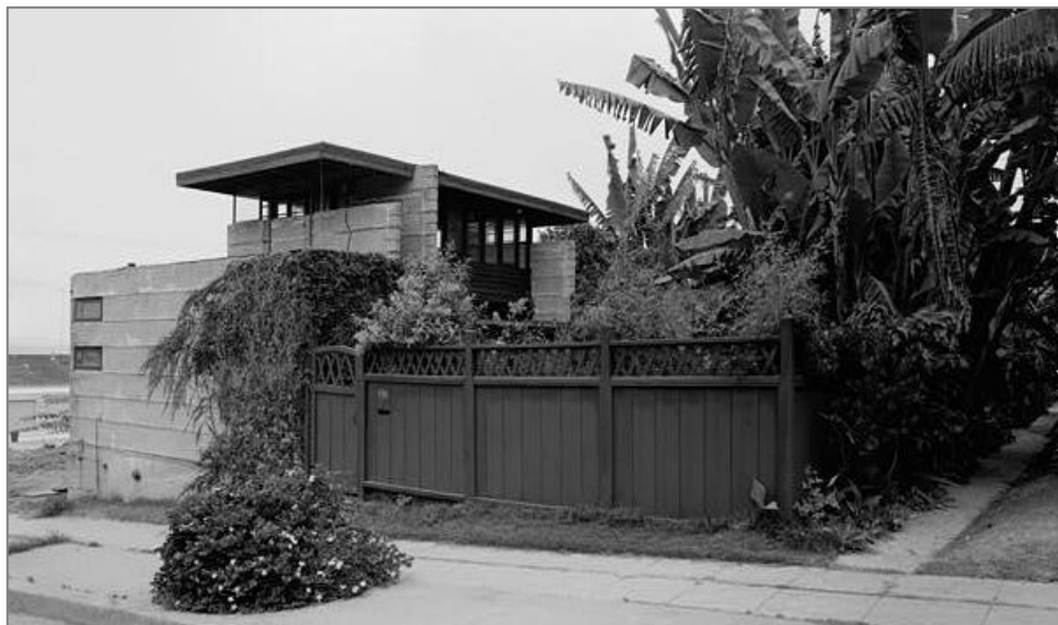
Figure 135. Pueblo Ribera Court, Rudolph Schindler (Library of Congress).
