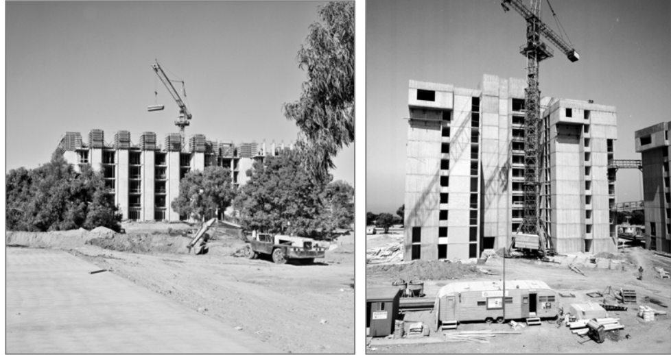
Figures 25-26. Muir College under construction, 1968-1969 (UC San Diego Digital Library Collections).
