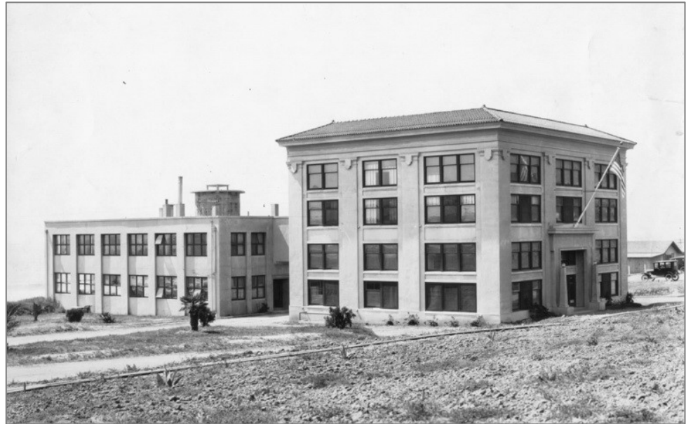
Figure 43. The Library-Museum Building (right), adjacent to Old Scripps (left), 1923 (UC San Diego Digital Library Collections).
