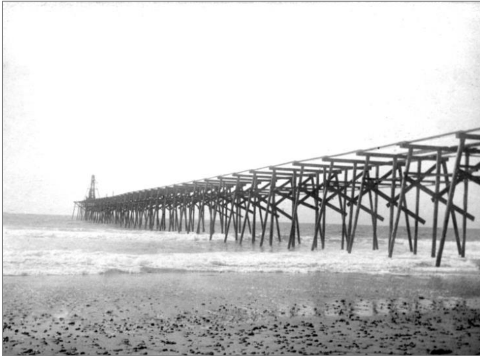
Figure 42. Scripps Pier under construction, 1915 (UC San Diego Digital Library Collections).
