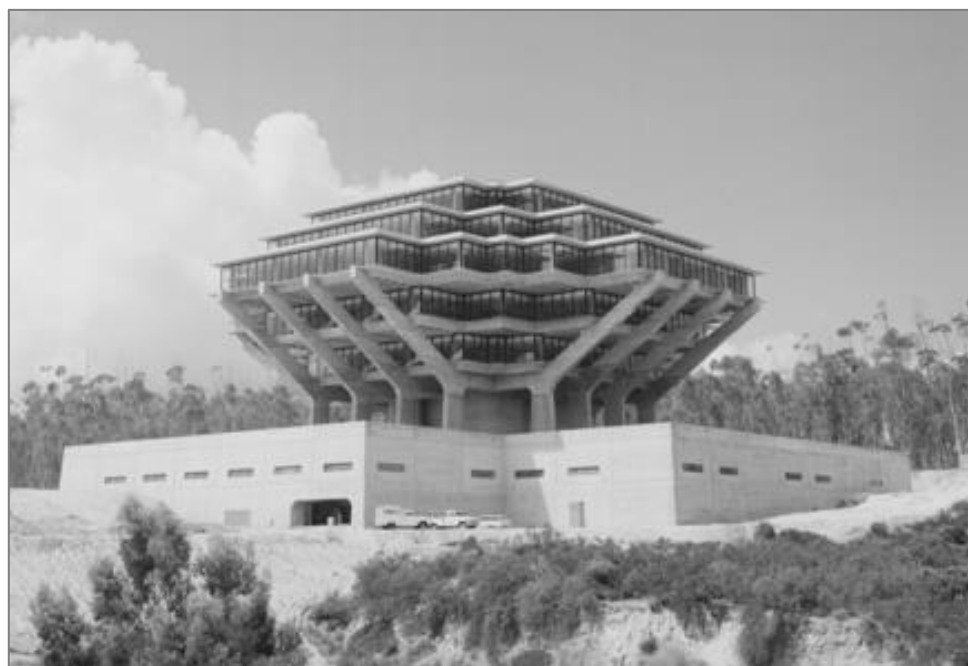
Figure 137. Central University Library (now Gessel Library), an iconic example of Modern architecture, 1970 (UC San Diego Digital Library Collections).
