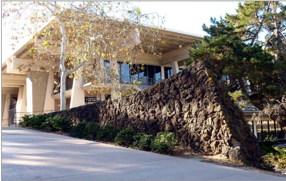
Figure 124. Lava rock retaining wall in front of Galbraith Hall, 2015 (ARG).
