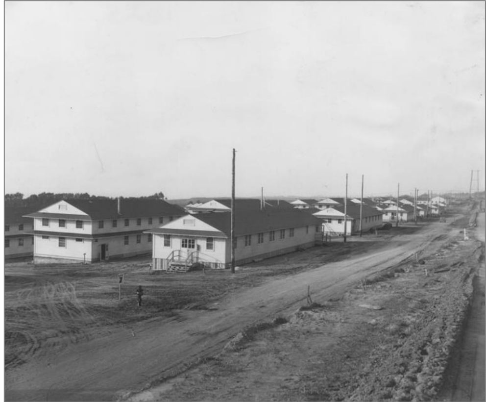
Figure 55. Buildings at Camp Callan, designed by Myron Hunt and H.C. Chambers, 1941 (Los Angeles Public Library Photo Collection).
