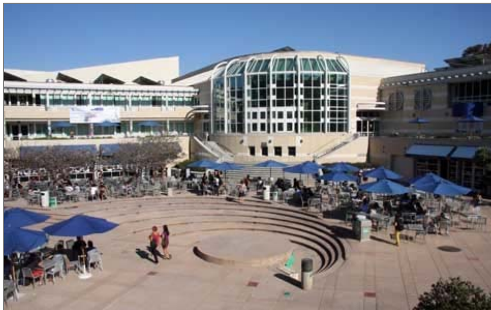
Figure 35. Price Center West, constructed 1989 (UCSD University Centers).
