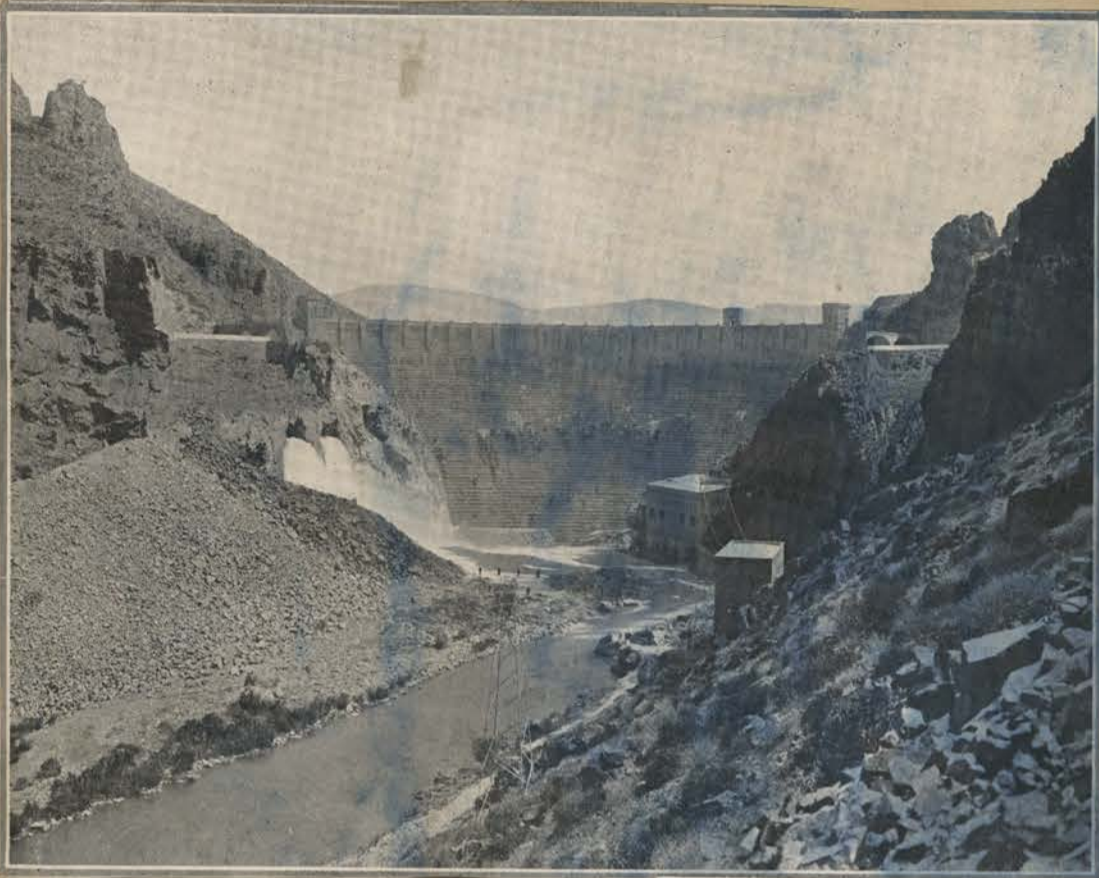
The big dam at Roosevelt checks and stores the waters of the Salt River and Tonto Creek, and in proper quantities allows it to return through the sluice gates to the bed of the river, where it flows on, taking up in its course the waters of the Verde River, and then heading for the diversion dam at Granite Reef. Here the flow of the three united streams is turned into great canals on the north and south banks of the river. The Granite Reef Dam is one of the largest weir dams in existence. It is thirty-eight feet from base to crest, and 1,100 feet long.
