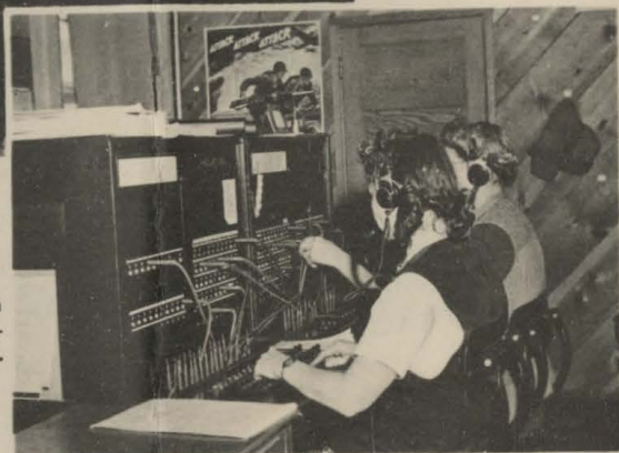
NERVE CENTER . . . civilian employees alternate with soldiers operating switchboard.
