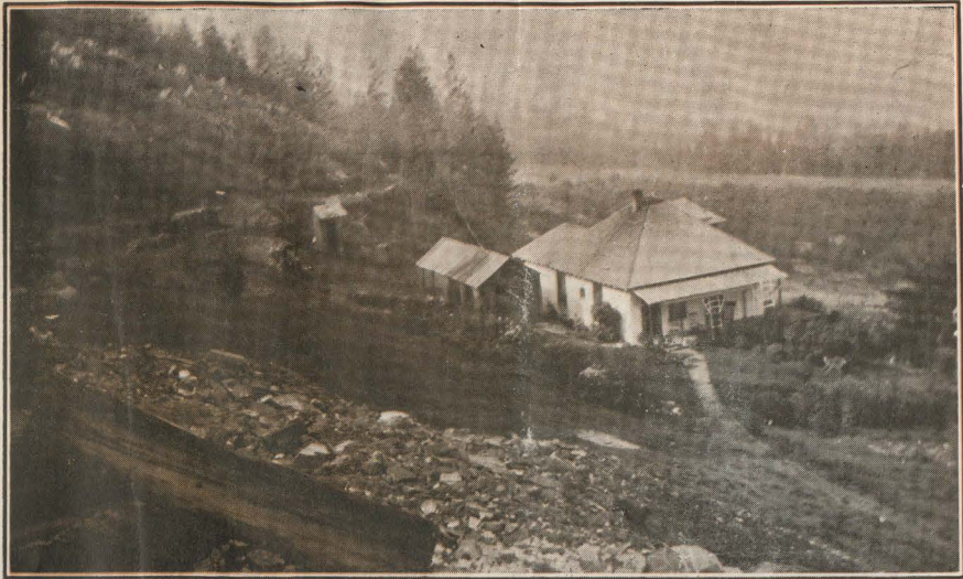
View of Boarding House.
