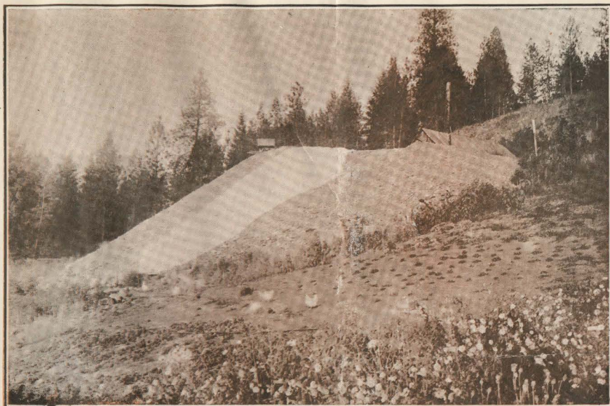
View of Main Dump.
