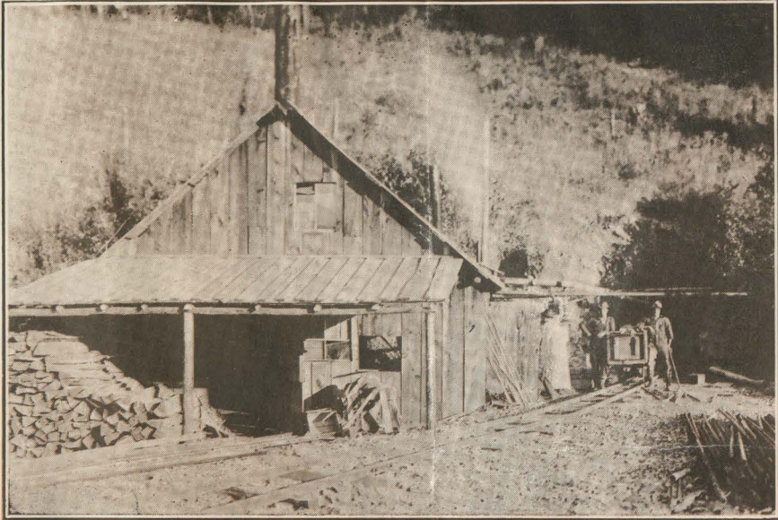
View of Engine and Boiler House at Portal of Main Tunnel.
