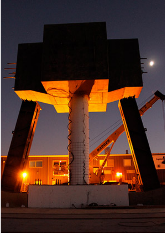
Engineers tested a 24-foot bridge column on the NEES @ UCSD shake table in September 2010.
