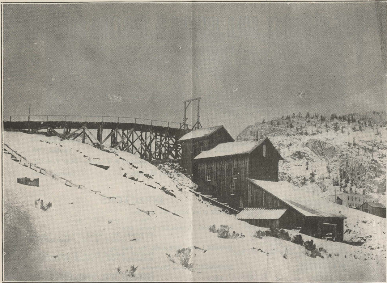
MILL OF SECURITY GOLD MINING AND MILLING COMPANY.
