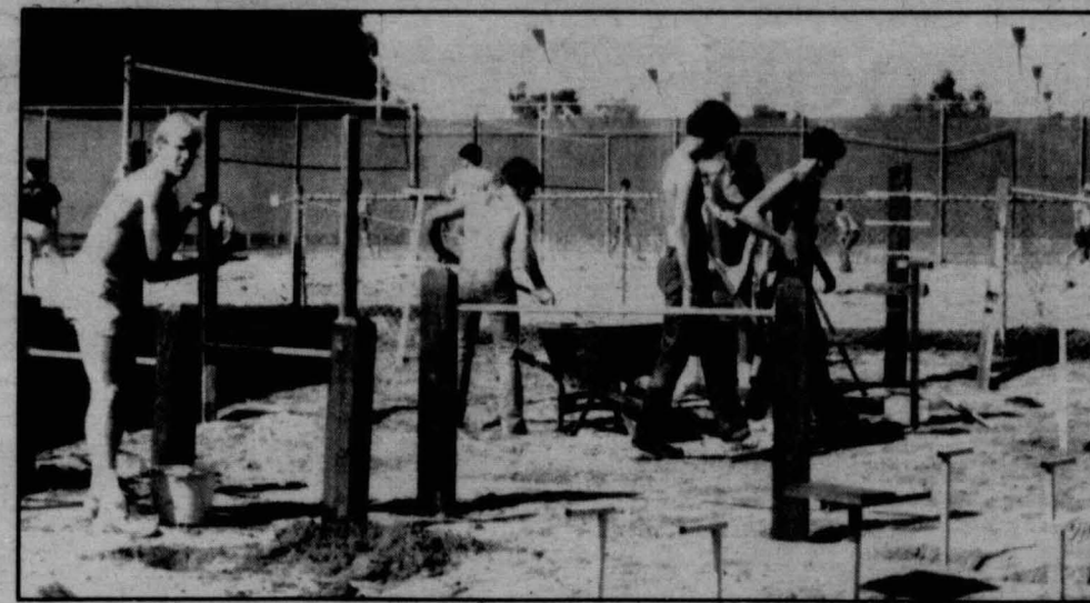
Members of the Phi Delta Theta fraternity hauled sand and constructed the stations for the Fitness Court, which opens today.
