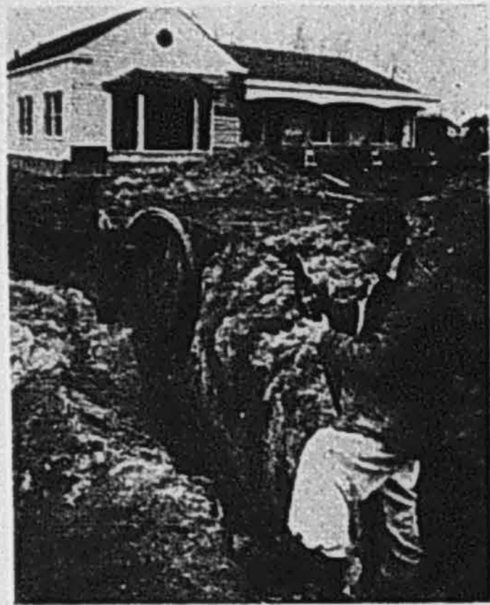
Flexible plastic pipe, sold in coils like this, eliminates the need for many fittings, thereby slashing installation costs.
