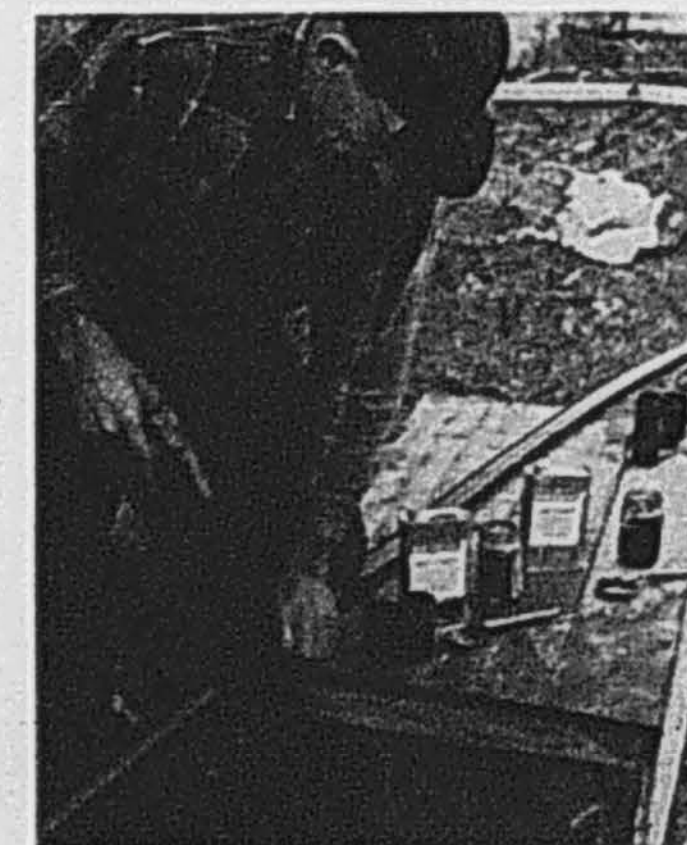
No expensive tools are needed to install plastic pipe. Pipe can be cut with any good hand saw, joined with fittings that are sealed with pipe cement.
