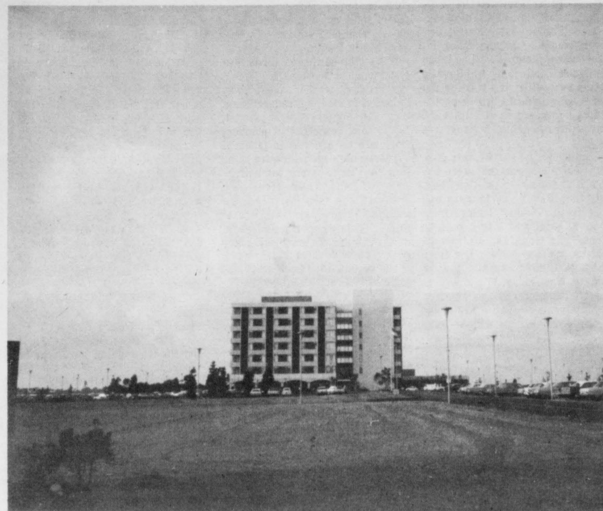
The 600-bed County-University Hospital above is currently operated by the School of Medicine and will be supplemented by a 350-bed University Hos-
