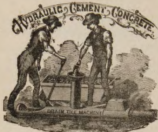
[Machine used for Making Continuous Concrete Pipe.]
