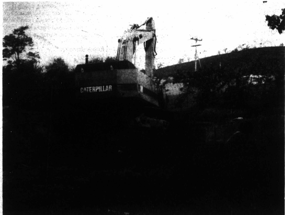
•Wanpela doza bilong Bee Construction Kampani i wok long klinim dispela hap ples we ol bai mekim dispela nupela haus bilong ol kompluta netwok bilong Works Dipatmen. Dispela em long Walgan.
