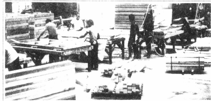
Components for the Fletcher designed 'Esi-build' modular housing system being manufactured in Port Moresby.
