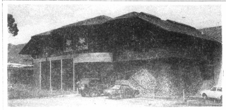
Coffee Industry Board headquarters and warehouse complex at Goroka
