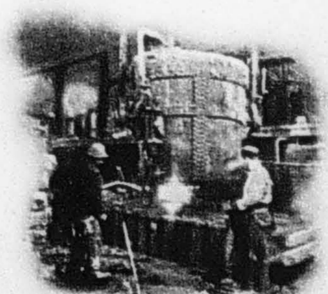
Pouring in Molds
