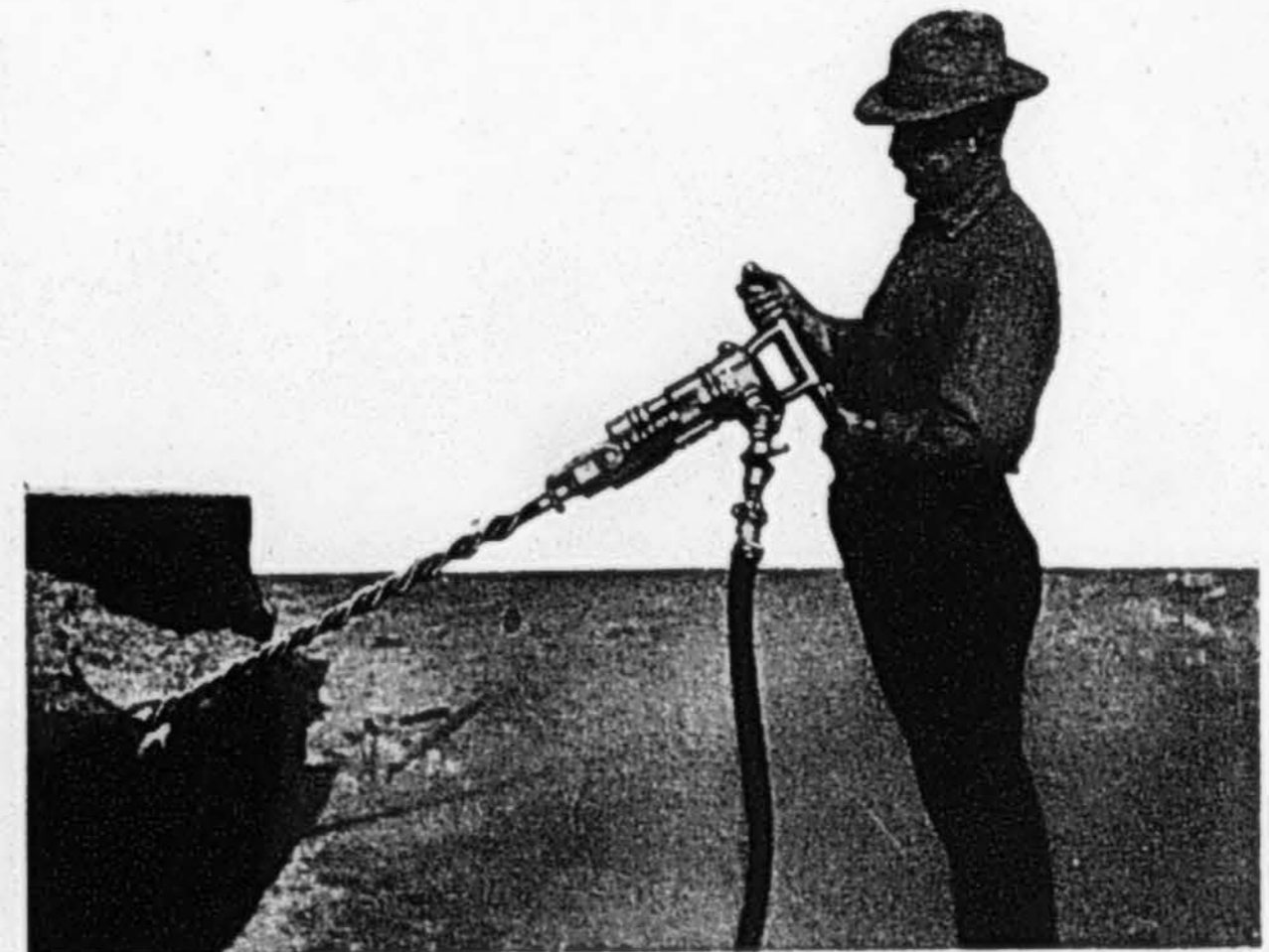
A66 "LITTLE HUMMER" Drill with auger bit as shown above is used for drilling ore, coal, sandstone, etc.
