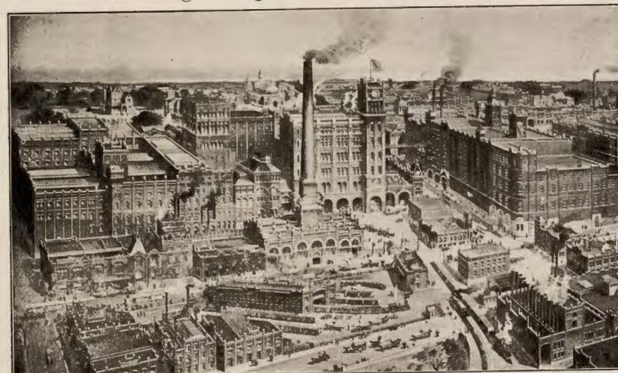
Principal Buildings of the Anheuser-Busch Brewing Plant, St. Louis, Mo., U. S. A.
