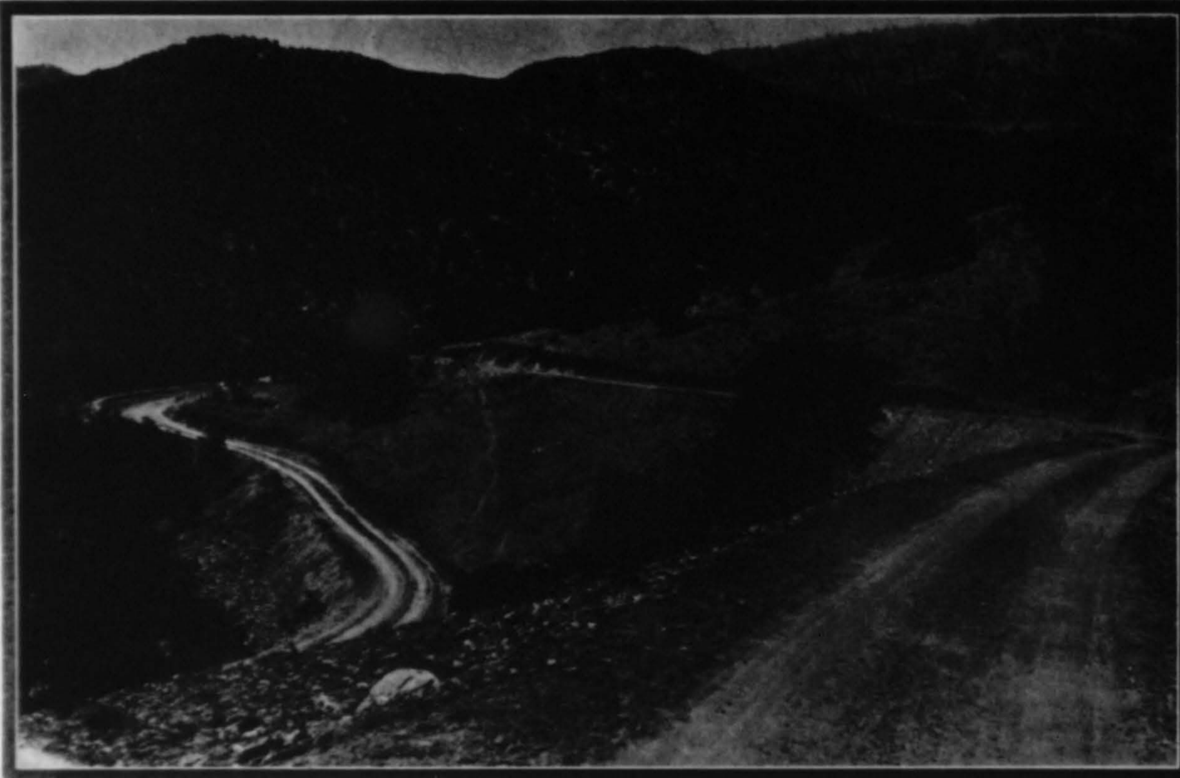
A well-constructed forest road in Arizona. The topography of the country necessitates a devious location
