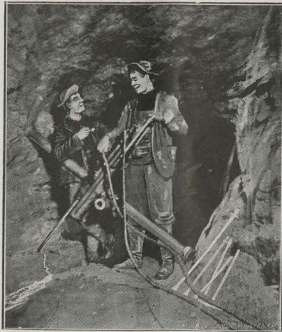
Leyner Air Compressor Drill Working on Breast of Tunnel
