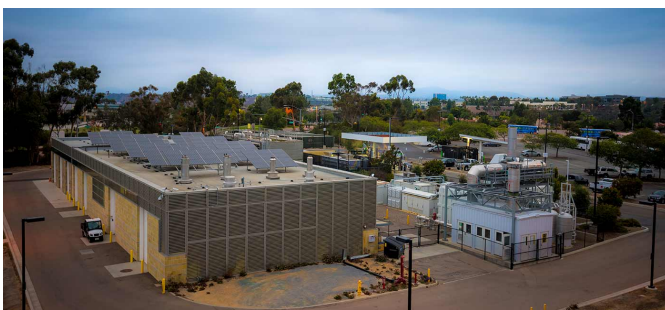
The UC San Diego microgrid, one of the most advanced in the world, is powered by a mix of on-site sources including a biogas-powered fuel cell and solar panels.
