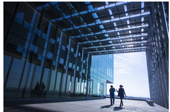
Solar panels on UC Merced's Science and Engineering Building, courtesy UC Office of the President
