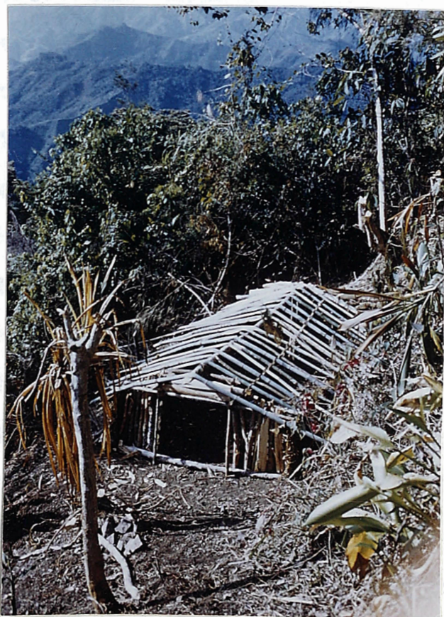
PLATE 2 MEN'S HOUSE UNDER CONSTRUCTION BY WABI AT KWIOP.
