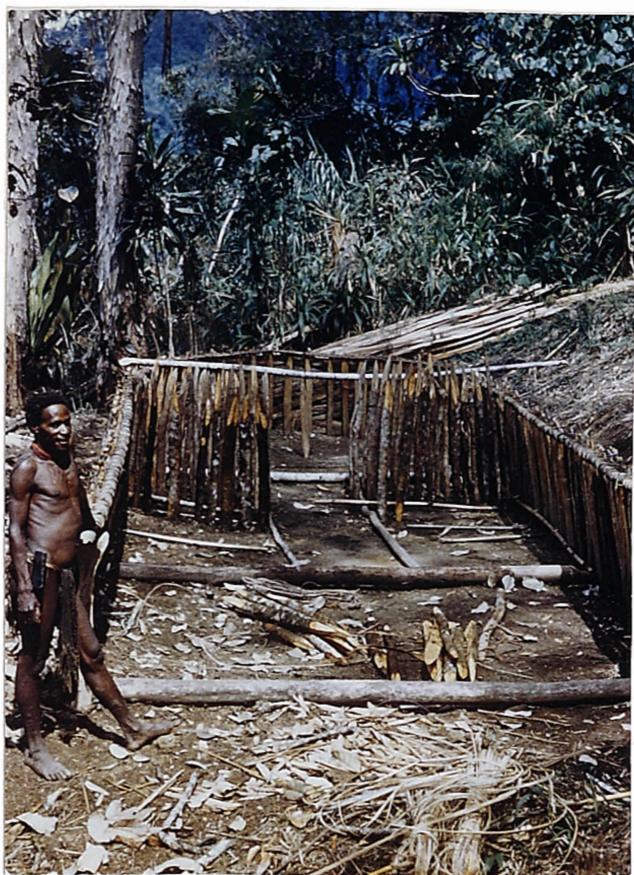
PLATE 1 WOMAN'S HOUSE UNDER CONSTRUCTION BY TSAPINDE. THE THREE DIVISIONS OF THE INTERIOR OF THE HOUSE ARE EASILY SEEN.
