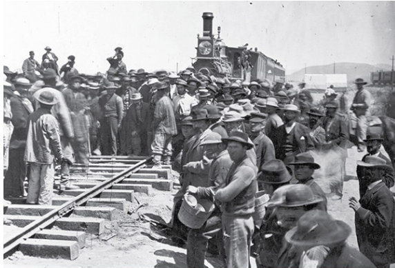
Chinese laying the last rail on May 10, 1869. Photo taken by Andrew J. Russell (1830-1902), a photographer assigned to document construction of the first transcontinental railroad as it stretched westward across the continent in the late 1860s. Photo by courtesy of the Kyle Watt Collection
