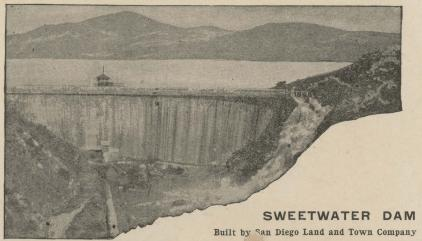
Length at base . . 76 feet. Thickness at base . . 46 feet. Height of dam from bed-rock . . 96 feet. Length at top . . 396 feet. Thickness at top . . . 12 feet. Reservoir Covers . . . . . . . . . 700 acres Solid Granite and Portland Cement. Forming lake three miles long by two miles wide.
