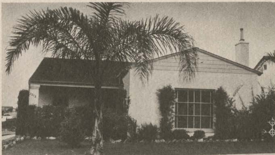
Plan 5974 Convenient front kitchen and compact arrangement in a modified California Monterey feature this plan Estimated monthly payment Including lot—FHA $32.38
