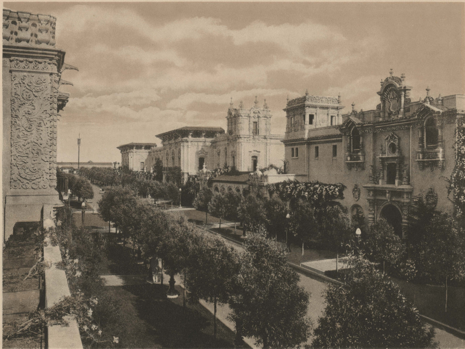
El Prado showing Commerce and Industries Building.
