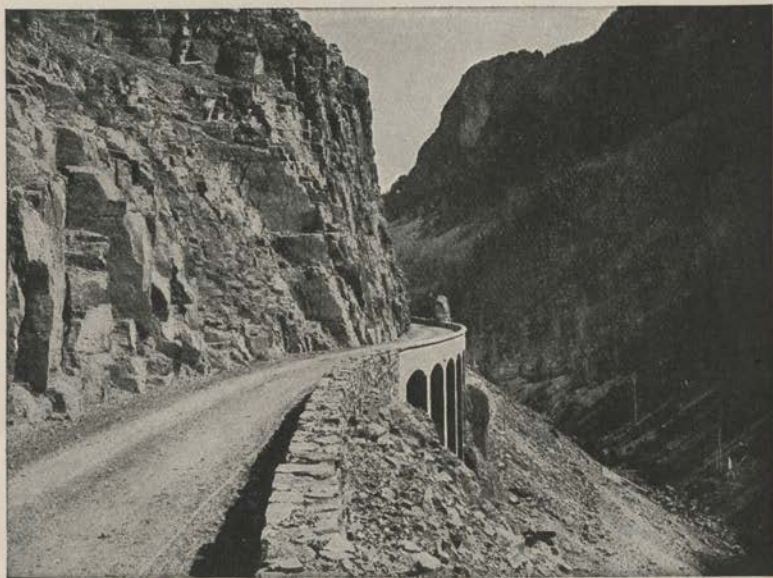
Golden Gate Canyon, between Norris Geyser Basin and Fort Yellowstone, has been improved by the Government with a Massive Concrete Viaduct.
