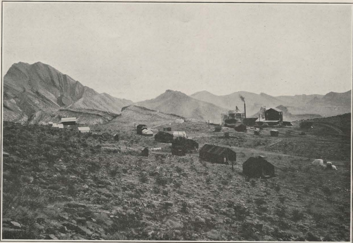
GENERAL VIEW OF PLANT AT MINE.
