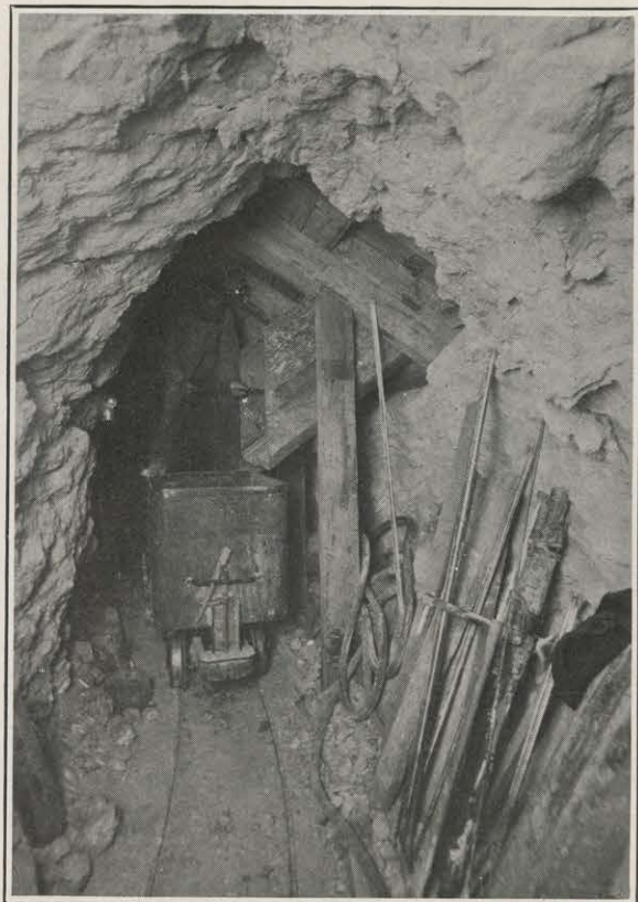
LOADING CARS WITH BORATE ORE FROM CHUTES IN THE MINE.
