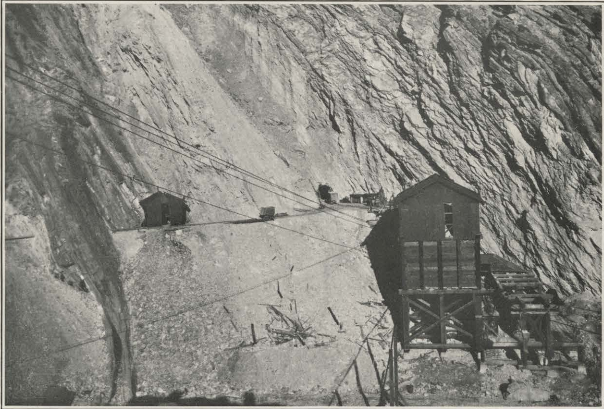
ORE BIN AND LOWER TERMINAL OF TRAMWAY AT THE MOUTH OF THE TUNNEL.
