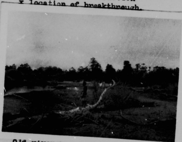
Old river bed showing first flow after work on fences.
